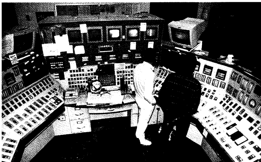
3. El Segundo station , built in 1955, has pioneered multivariable control technology. In a project completed last summer, El Segundo backfit the technology for the historically tough challenge of steam-temperature control in a reheat steam cycle in Units 3 and 4
