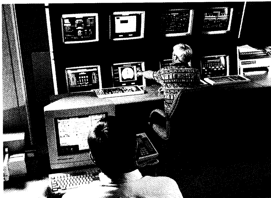
4. Bergen station operators updated a 1960s-vintage control system and found that a simulator can streamline backfit projects. Engineers originally ordered the simulator for operator training, but also used it to identify construction errors before commissioning
